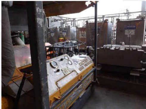
Umbilical Monitoring, Testing, and Commissioning: Specialized personnel and equipment to complete job specific requirements for an efficient offshore installation campaign
