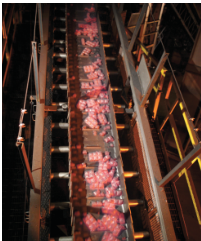
Top: Conveyors carry iron fines and coal into the plant for processing; refined iron exits from the buildings housing the furnaces. Iron Dynamics' location next to SDI's Butler flat-roll mill allows quick, convenient transport of HBI or ladles of hot, liquid pig iron to the steel mill's melt shop, which is at the right edge of this photo. Bottom: Hot-briquetted iron (HBI) produced by Iron Dynamics serves as a lower-cost substitute for purchased steel-scrap and pig-iron ingots in SDI's steelmaking process.
