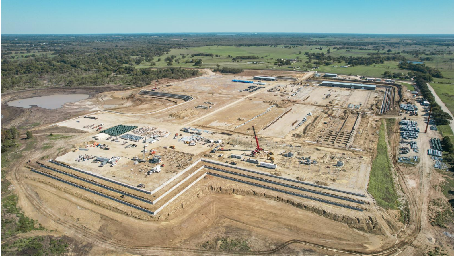
Corsicana Facility Under Development October 31 st , 2023
